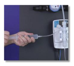
**Step 58:** Using the syringe kit, slide the syringe onto the air bleed barb and draw the plunger back. Chemistry should enter the syringe. Eject the chemistry from the syringe into the chemical bucket.
