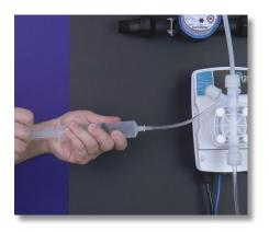
**Step 84:** Using the syringe kit, slide the syringe onto the air bleed barb and draw the plunger back. Chemistry should enter the syringe.
